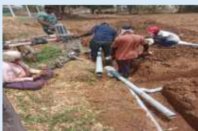
Members supervising underground pipeline installation
