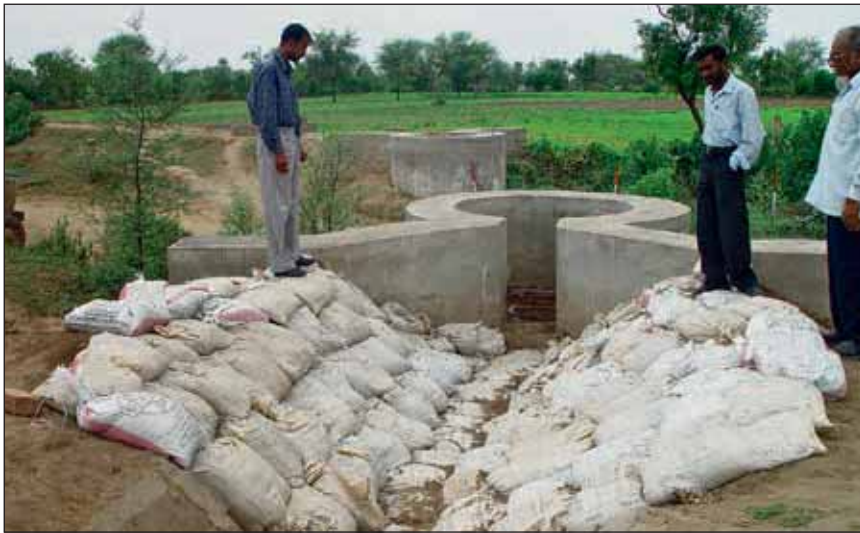
Sometimes canal water over topping causes damage to distribution network
