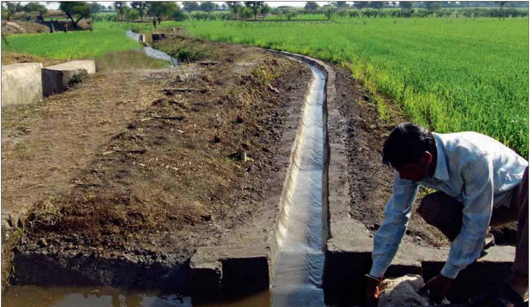
Field channel constructed in MP project for reducing the wastage of water at farm level
