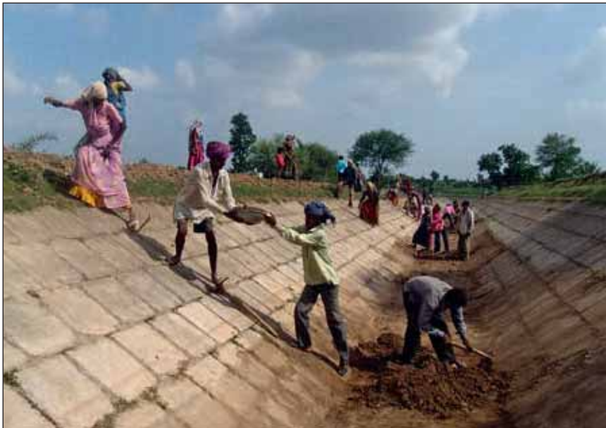
Farmers identified that at some places, the canals got heavily silted and therefore its water carrying capacity was reduced
