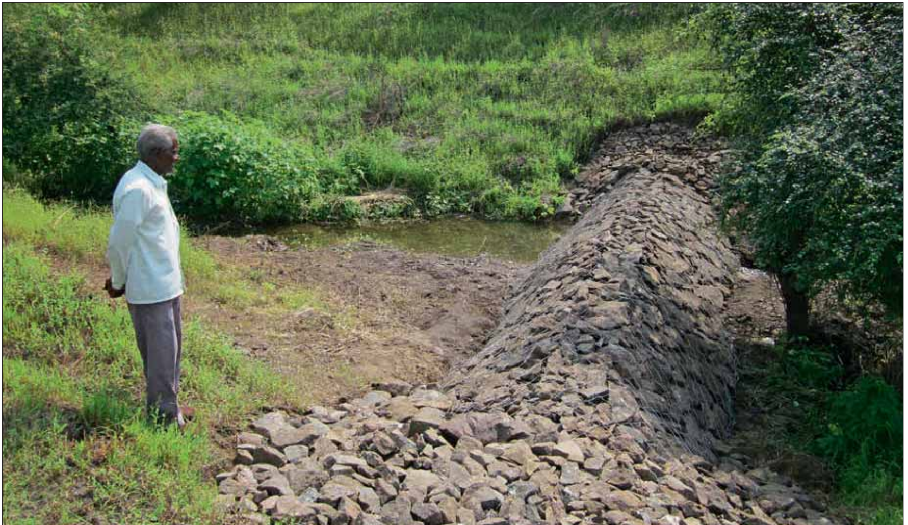
The water user group member constructed gabion on his land to prevent soil erosion
