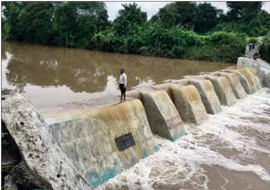
The villagers closed the gates of check dam to harvest water after monsoon on Lodhari River- Integrated Watershed Development Project, Dewas, MP
