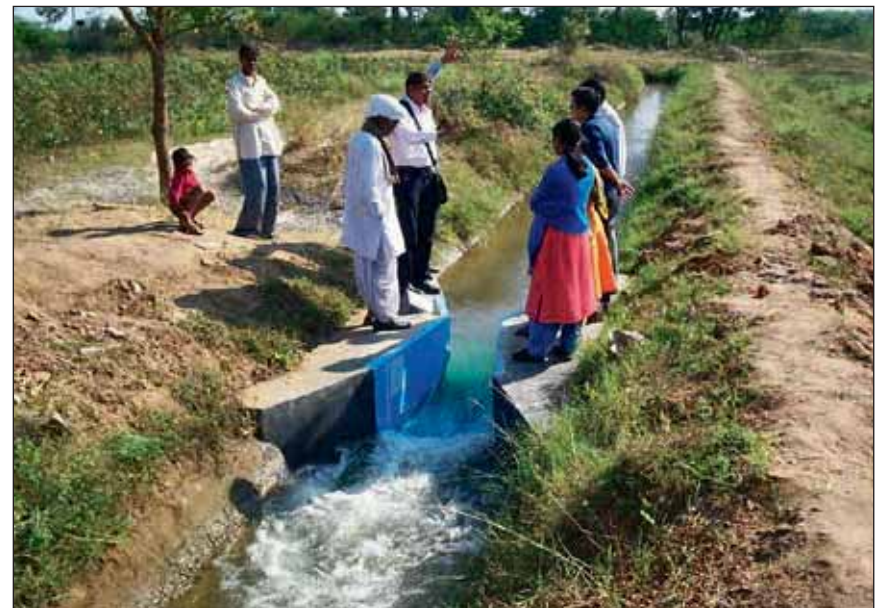
Every drop of water counts-volumetric structure fixed by WUA on their canal for measuring water used for irrigating their land
