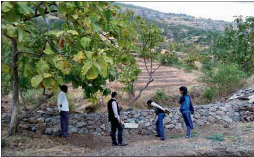
A small barrier has been built on the hill top to protect precious land from degrading
