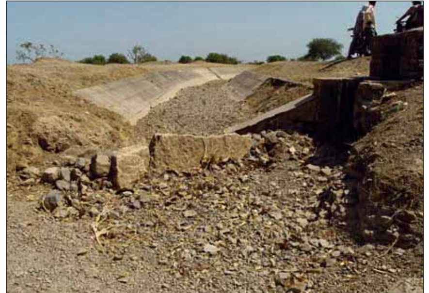
The unlined sections get eroded due to flood and improper maintenance causing tail end deprivation
