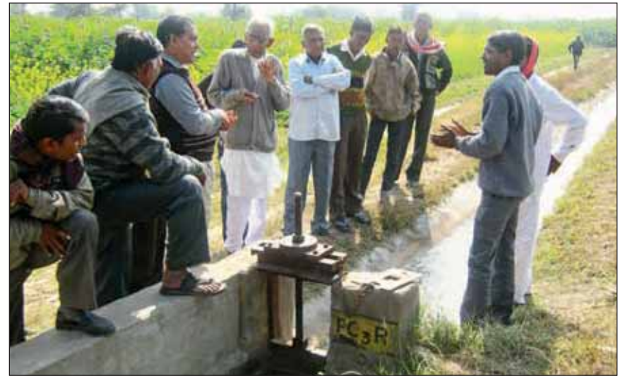
The WUA revived control gates for rotational supply of water to all farmers
