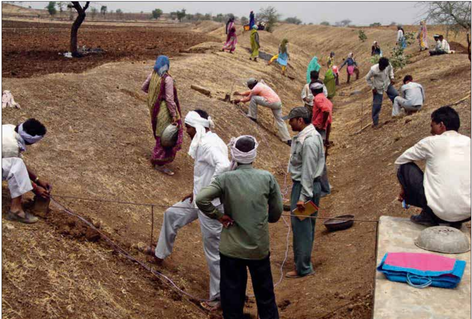
Recapacitating canals for better water supply-Canal reshaping work under progress in Jobat irrigation project, MP
