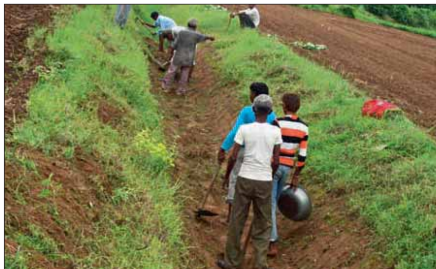
Desiltation of canals by WUAs in Man Project, MP
